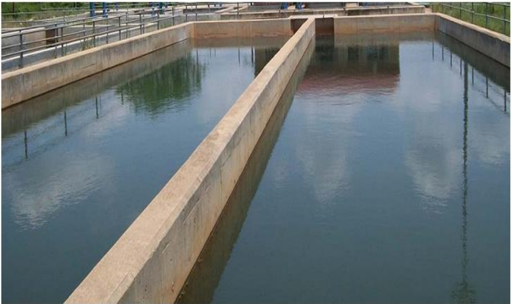
Fig. 1: Rectangular horizontal flow sedimentation tank
